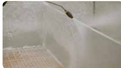
STEP 4 Rinse with water (high pressure cleaner) and let dry
