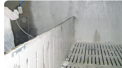
STEP 2 Apply gel with high pressure foam lance (50-150 bar).
