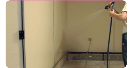
STEP 3 Rinse with water Medium or high pressure cleaner (25-150 bar, 12-30L/min.) and let dry.
