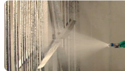
STEP 2 Foaming With high pressure after every hatch (dosage 1%).
