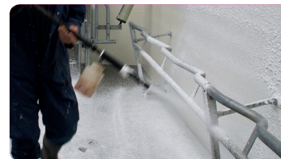
STEP 2 Apply foam or spray with high pressure foam lance (50-150 bar).
