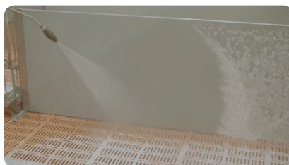
STEP 4 Cleaning with high pressure water jet (50-150 bar).
