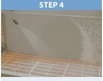
Cleaning with high pressure water jet (50-150 bar).
