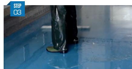
STEP 03 Rinse with water Rinse with water (high pressure cleaner (50-150 bar and 12-30 Ls per min) and let dry.
